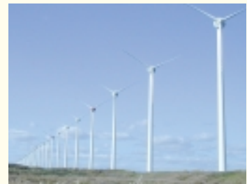
Horonobe Wind Power Generation's Otonrui Wind Power Plant.
